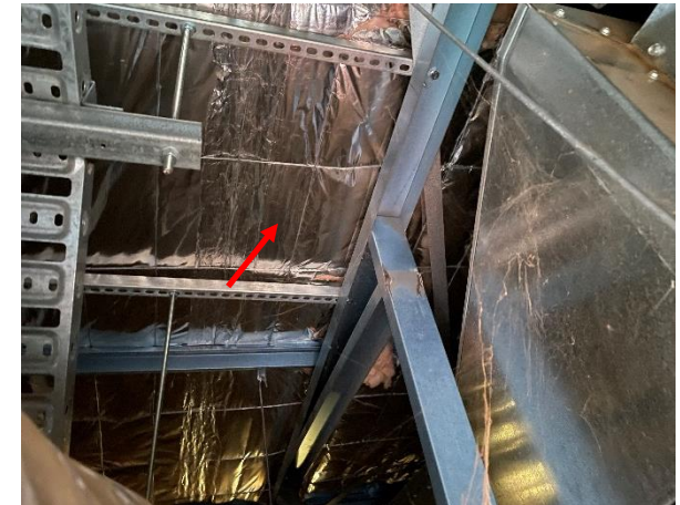
Photo 24: Throughout Mental Heal Unit interface, ceiling cavity underside of roof – Assumed SMF sarking
