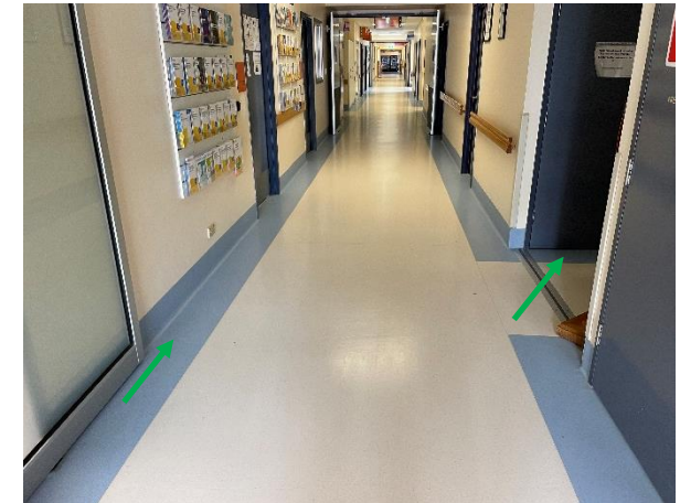
Photo 15: Oncology unit and mental health service office corridor, floor – blue speckled vinyl sheeting
