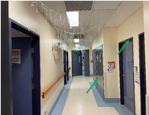
Photo 22: Throughout mental health unit interface, doors and door frames – Non-lead based blue paint
