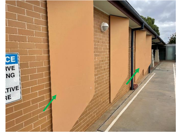
Photo 3: Oncology Ward, external window covers – Non-asbestos containing compressed fibre cement sheeting
