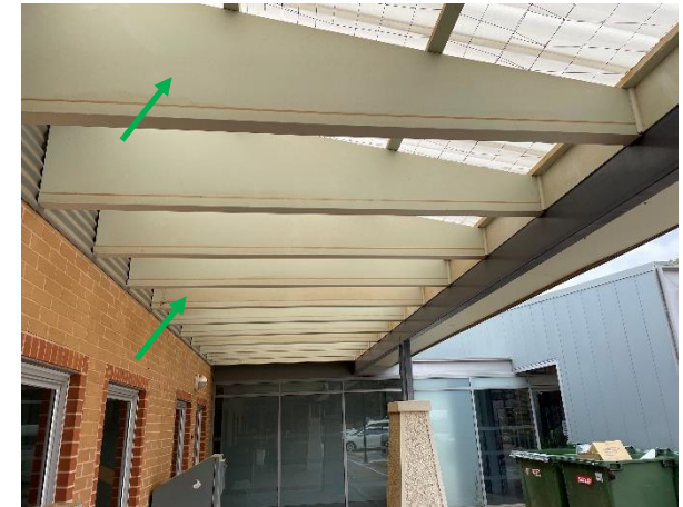
Photo 6: West of mental health service office, box cover to rafters of awning – Non-asbestos containing fibre cement sheeting
