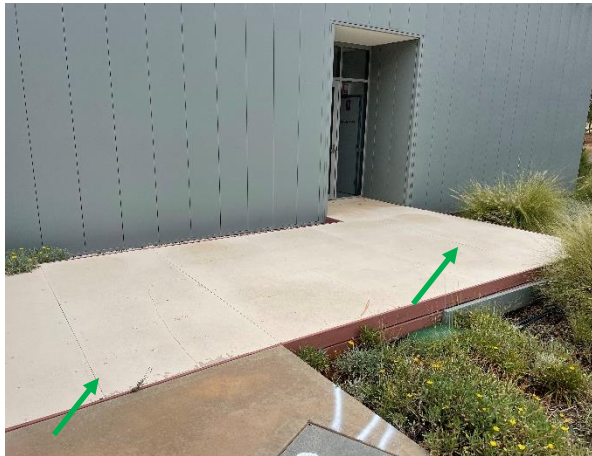
Photo 10: Sub-acute rehabilitation unit northern entrance way, floor – Non-asbestos containing compressed fibre cement
