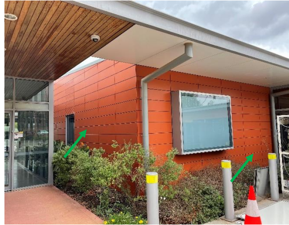
Photo 8: Sub-acute rehabilitation unit, external wall cladding – Non-asbestos containing compressed fibre cement
