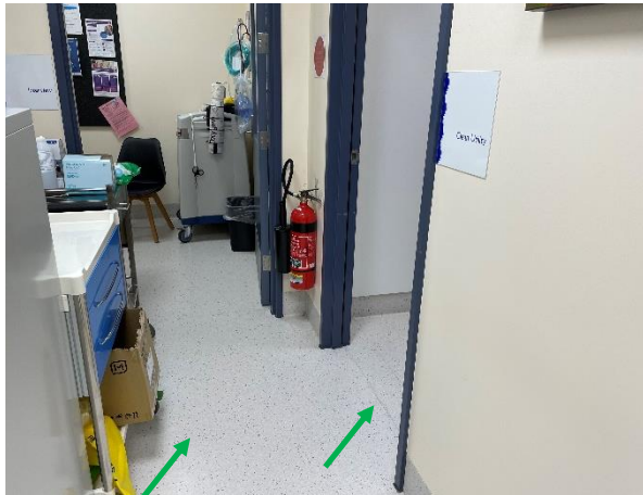
Photo 13: Oncology unit and mental health service office, floor – Non-asbestos containing grey speckled vinyl floor sheeting
