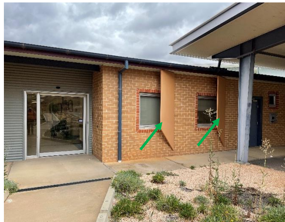
Photo 29: Emergency department, external window covers – Non-asbestos containing compressed fibre cement sheeting
