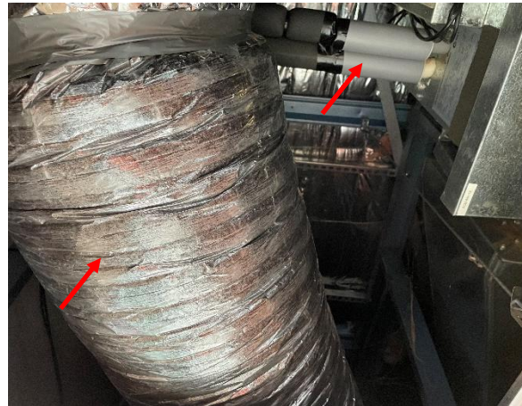
Photo 26: Throughout Mental Heal Unit interface, ceiling cavity ducting and pipework – Assumed SMF insulation
