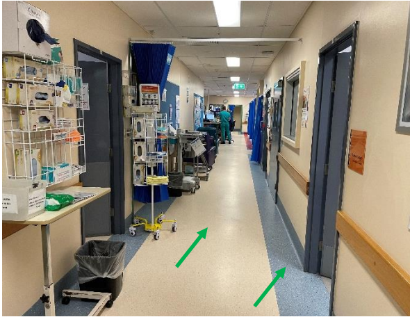
Photo 31: Emergency department, internal floors – Assumed non-asbestos containing beige and blue speckled vinyl sheeting
