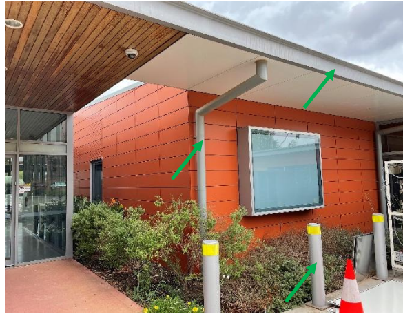
Photo 20: Sub-acute rehabilitation unit, external steel frame, down pipes and bollards – Non-lead based grey paint
