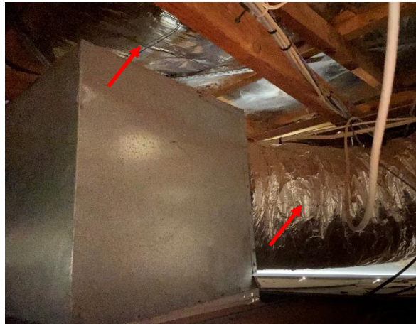
Photo 35: Emergency department, ceiling cavity – Assumed SMF sarking and ducting
