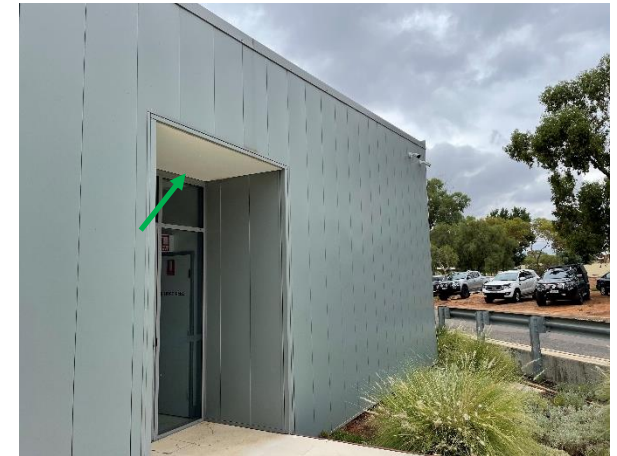
Photo 12: Sub-acute rehabilitation unit northern entrance way, soffit lining – Non-asbestos containing compressed fibre cement
