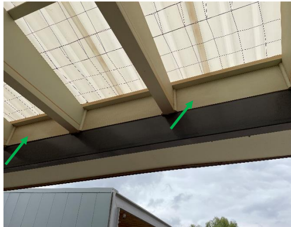
Photo 5: West of mental health services office, external awning infill panel between awning roof and eaves – Non-asbestos containing fibre cement sheeting
