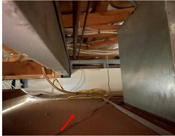
Photo 32: Emergency department ceiling cavity – elevated levels of lead within settled dust, it is noted this dust does not contain asbestos
