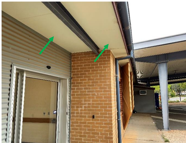
Photo 28: Emergency department, external eaves – Non-asbestos containing fibre cement sheeting
