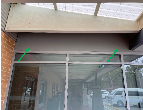
Photo 7: Southern external gill wall of corridor to sub-acute rehabilitation unit and roof, infill panel – Non-asbestos containing fibre cement sheeting
