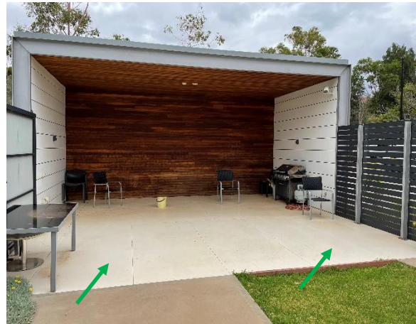
Photo 11: BBQ area, floor – Non-asbestos containing compressed fibre cement
