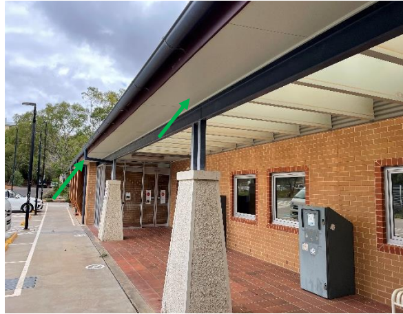
Photo 2: Oncology Ward, external eaves – Non-asbestos containing fibre cement sheeting
