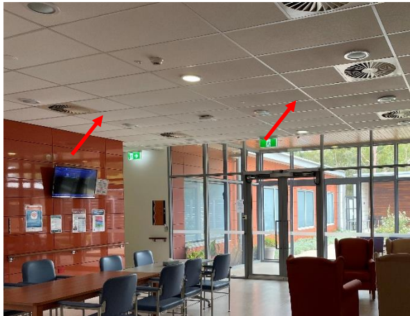
Photo 25: Throughout Mental Heal Unit interface, ceiling – Assumed SMF suspended ceiling tiles
