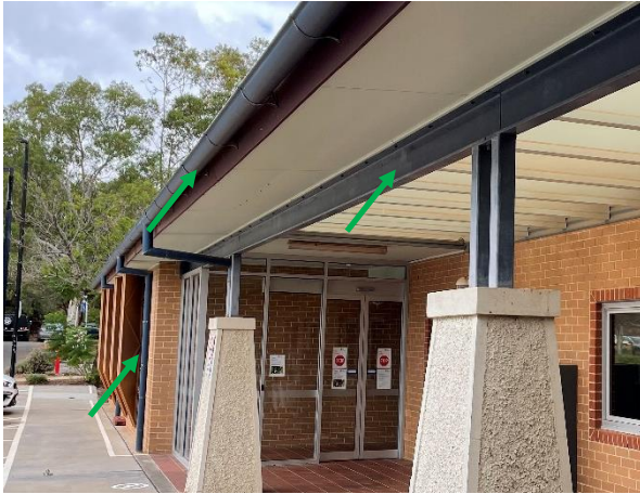
Photo 19: Oncology ward and mental health services offices, external downpipes, steel framework and I beams – Non-lead based blue paint
