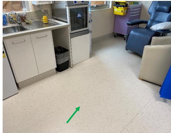
Photo 14: Oncology unit ward, floor – Non-asbestos containing white speckled vinyl sheeting
