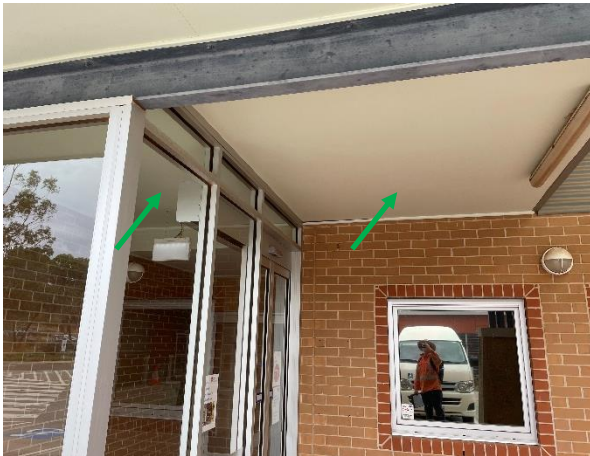
Photo 4: Oncology ward, western entrance way external and internal ceiling lining – Non-asbestos containing fibre cement sheeting
