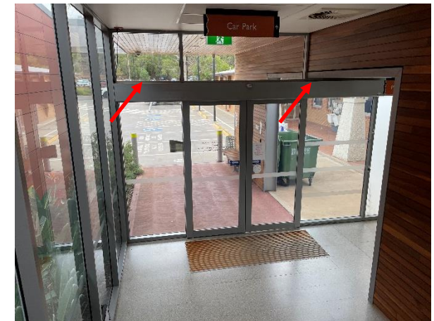
Photo 18: Corridor between mental health services office and sub-acute rehabilitation ward, atop sliding door motor housing – elevated levels of lead within settled dust, it is noted this dust does not contain asbestos
