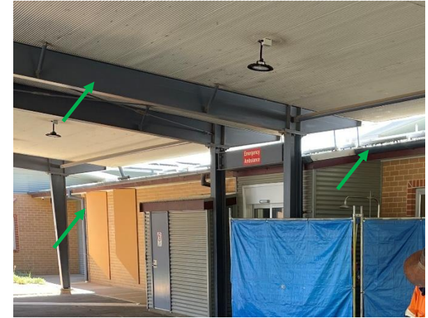
Photo 33: Emergency department, external downpipes, gutters and I beams External ground surface – Assumed non-lead based blue paint
