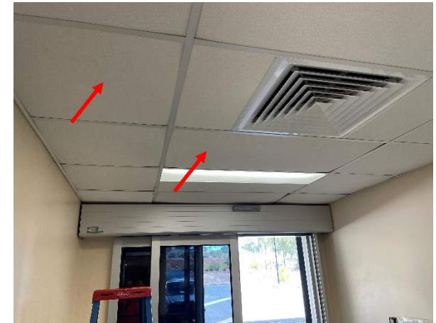
Photo 36: Emergency department, ceiling – Assumed SMF suspended ceiling tiles
