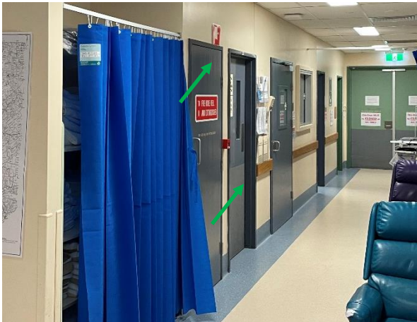
Photo 34: Emergency department, door and door frame – Assumed non-lead based blue paint
